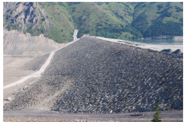
Photograph 2 (left) and 3 (right). Rough and loose surface configurations can be made using an excavator on slopes up to 2:1 or 26°. Large areas can be treated for a cost of about $700/ha.
