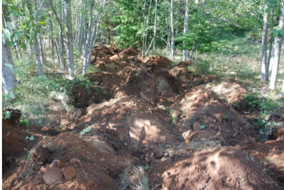
Photograph 4 (left) and 5 (right). Forest access roads and other small areas can be treated using the rough and loose technique (left) as well as areas with coarse substrates (right) such as this old dam site with alluvial boulders, cobbles and gravels.
