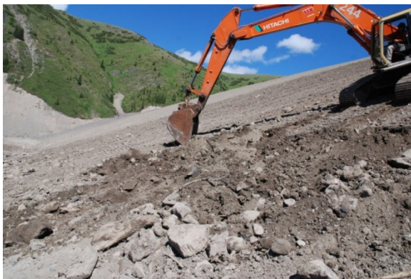
Photograph 2 (left) and 3 (right). Rough and loose surface configurations can be made using an excavator on slopes up to 2:1 or 26°. Large areas can be treated for a cost of about $700/ha.
