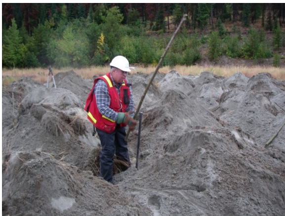
Photograph 6 (left) and 7 (right). Live staking in the rough and loose soils of this tailings pond is easy and allows the cuttings to grow rapidly (right, start of 2 nd year growth for cuttings)
